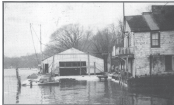
Original YYC Clubhouse at right - boat shed beyond was destroyed by a snow load .
