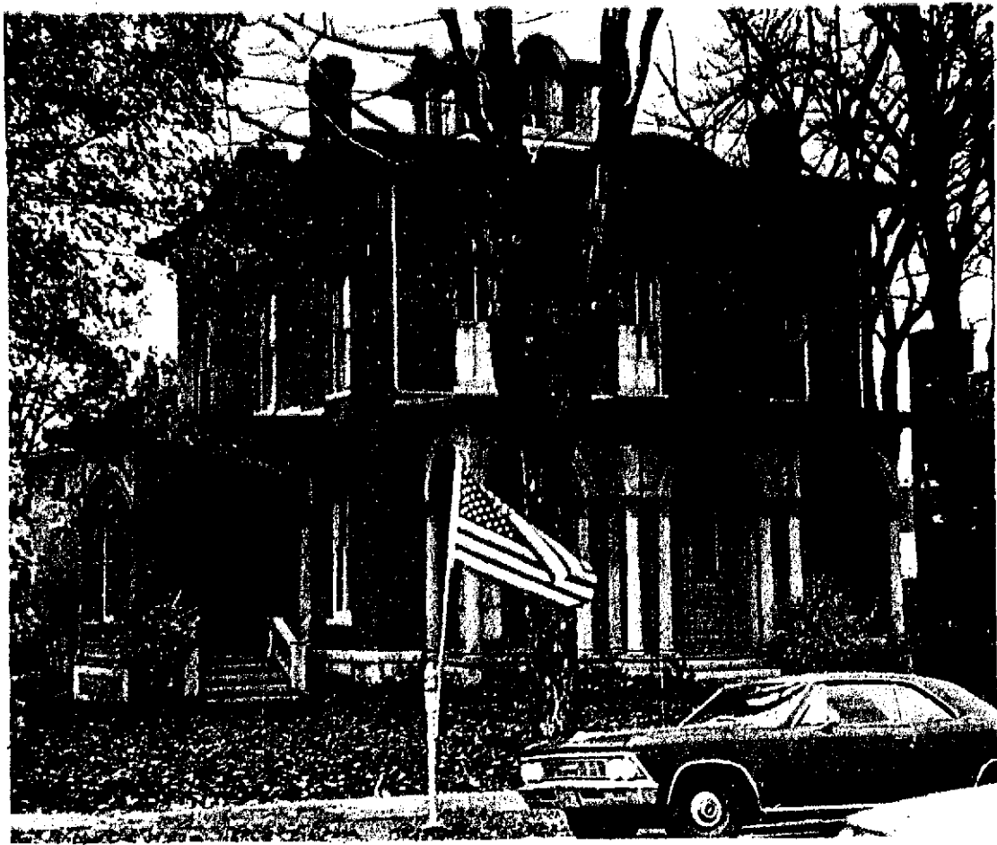
THE ABELL HOUSE, 429 Central avenue, Dunkirk.
