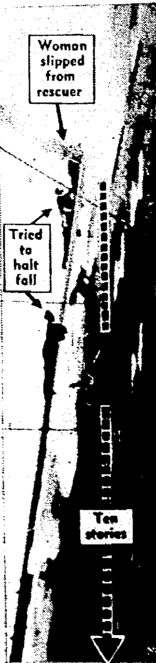
Choking in billowy clouds of smoke as she was carried down scaling ladder, Mrs. Travis Harrison lost her hold on a fireman's rock and dropped to her death. Fire gutting inside of Kansas City hotel necessitated outside rescue.
