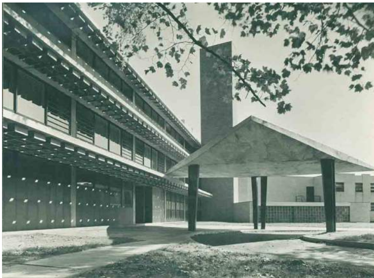
Figure 1: Photograph of Radbill addition to the Philadelphia Psychiatric Hospital circa 1953 (Source: The Louis I. Kahn Collection, University of Pennsylvania and the Pennsylvania Historical and Museum Commission).
