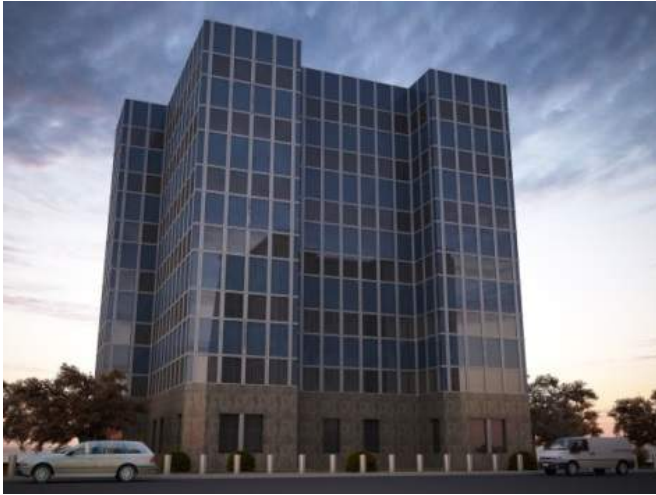
Figure 1: Example of an installation of the steel stud curtain wall described in the paper.
