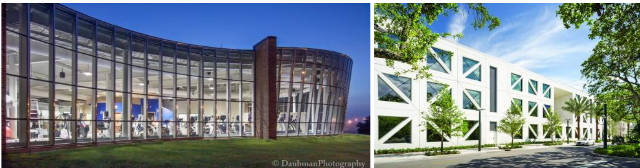
Figure 1: Project examples of the architectural design freedom offered by EC Glass. Left image: Butler County Healthcare and Rehabilitation Center, David City, NE, where EC glass was used to create a large, segmented sloped curtain wall that maintains large expansive views of the outside countryside and a comfortable day-lit interior to support faster patient recovery. This design would have been almost impossible to realize with conventional shading systems. Photo courtesy of Daubman Photography. Right image: The Frost School of music, Miami, FL, where EC glass was used in large triangular format to create a unique design that could not have been realized if exterior shading was used for sun control. Photo courtesy of Moris Moreno.
