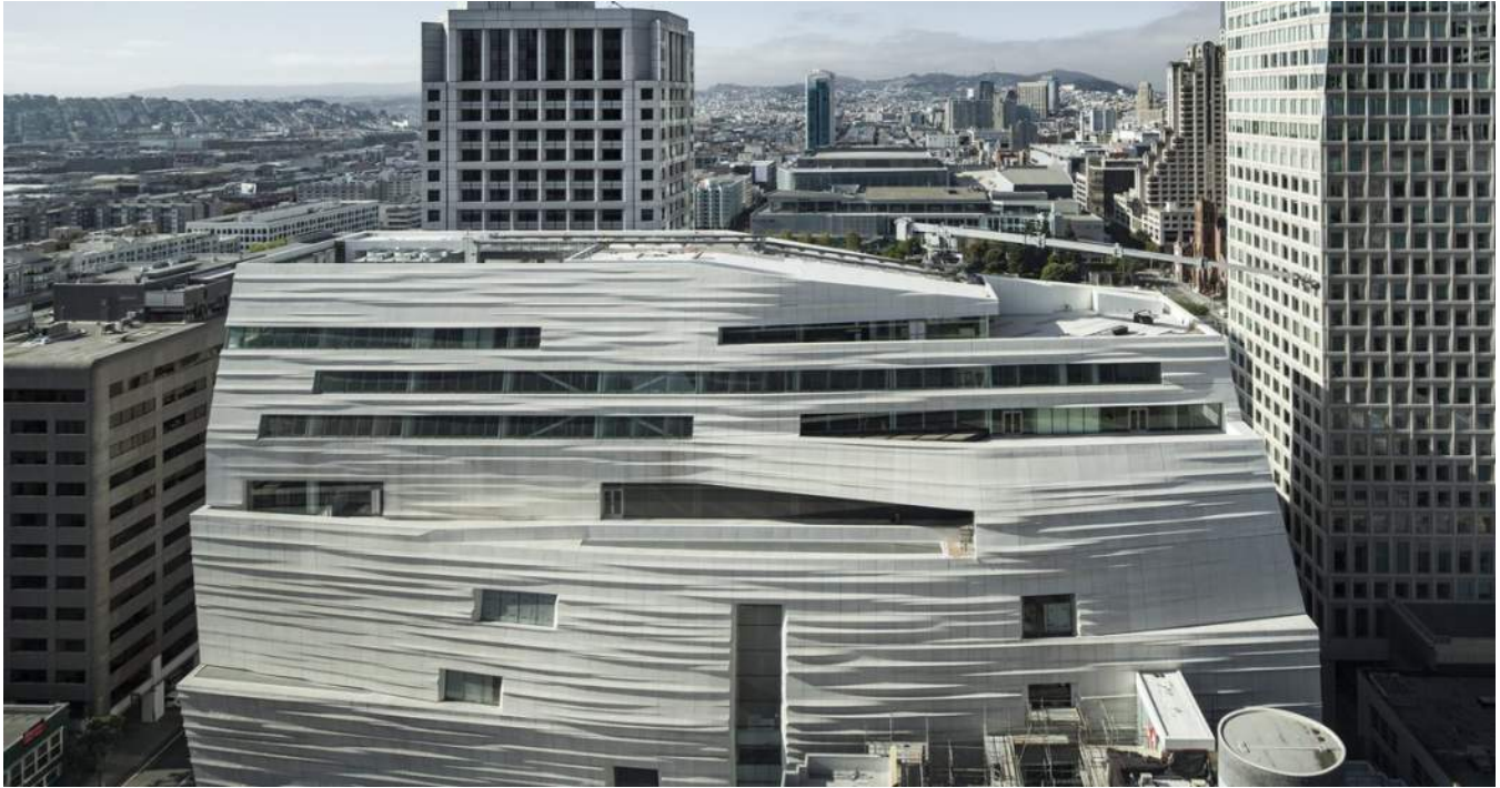
Figure 1: SFMOMA, an example of complex geometry realized using prefabricated panels, recently completed in San Francisco. Photo courtesy of Enclos.
