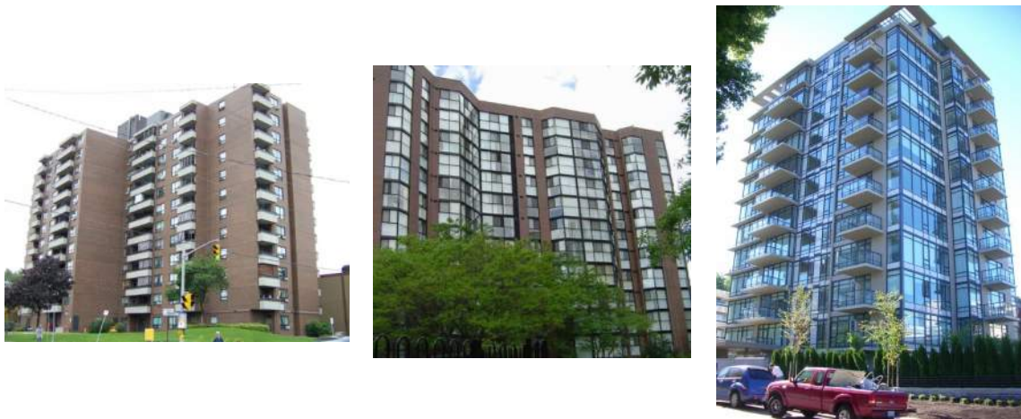
Figure 1: The evolution of Canadian window wall, from punch window (left) to the entire building envelope (right). All Photographs © Morrison Hershfield, 2106.
