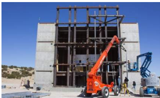
Test Reaction Structure
