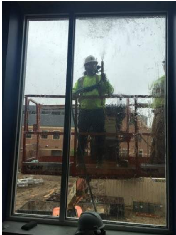
Figure 3: View of a field hose water test onsite
