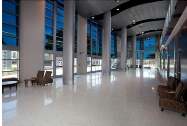
Figure 2: Interior view of the student services center at Chabot College, Hayward, CA. This highly glazed south facing atrium features EC glass on 3 sides and because of the peak load reductions provided, the architect was able to create a naturally ventilated space with no mechanical cooling.
