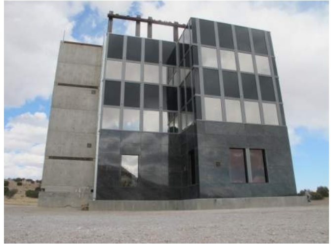
Figure 2: Full-scale test article and setup employed for blast tests.
