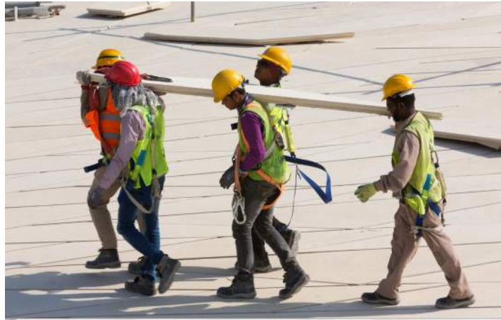
Figure 3 National Museum of Qatar – installation of panels.
