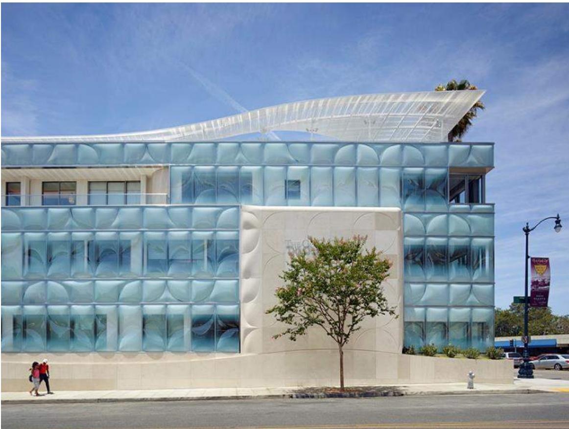
Figure 1: The glass in the façade of The Gores Group Headquarters in Beverly Hills, USA was the result of a close collaboration between the architect and several fabricators. The innovated material and production process was developed specifically for this project. (Photo by Bruce Damonte.)
