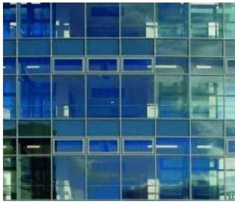
Figure 1: The aesthetical appearance of a shadow box in a curtain wall. Cork University Maternity Hospital, Cork, Ireland. Photo courtesy of Schueco Int. KG.
