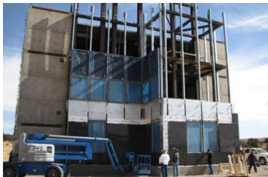
Figure 3: Installation of SSCW test structure: Installation of second floor cassettes
