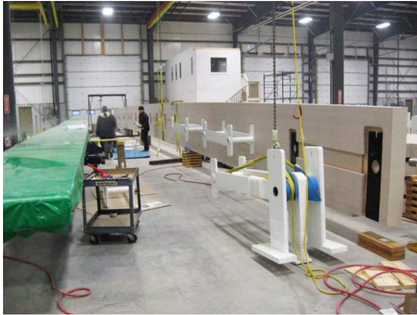
Figure 29. Factory production of the roof beams for the Kimbell Museum. The white painted pedestals were set on high precision bridge bearings. These bearings are in turn set on mounting pads that accommodated the location tolerances of the reinforced concrete walls. The beams were profiled and pocketed on a CNC router. (Photo by author)
