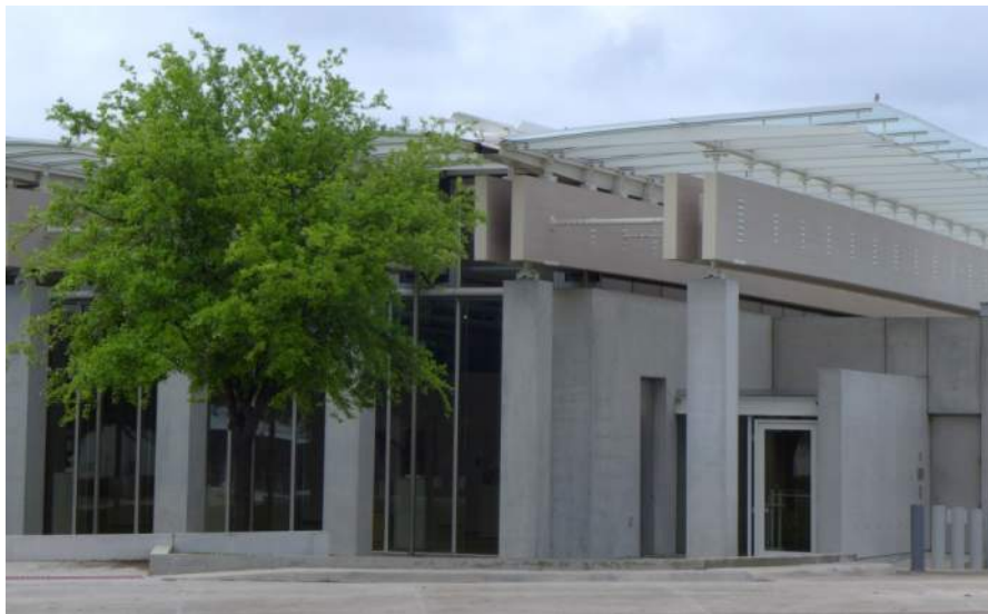
Figure 28 The Renzo Piano Building Workshop addition to the Kimbell Art Museum on Fort Worth, TX. The roof beams are 32M wood and metal composite Glulam beams. (photo by author)
