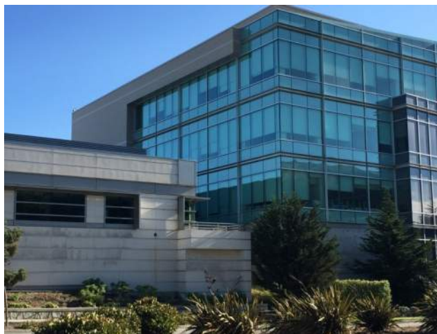
Figure 3: Typical sight of office building with shades down even when the sun is not directly on the façade. This photo was taken of the northeast corner of a building in San Francisco at 5pm in the afternoon. Most of the shades are pulled down over most of the window area even though the sun is on the other side of the building and has been for many hours.
