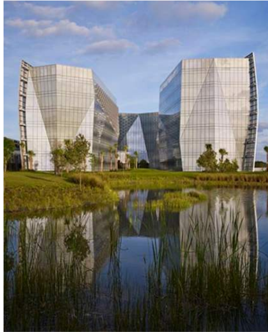
Figure 13: The completed Miramar building, with its restored site and geode form.
