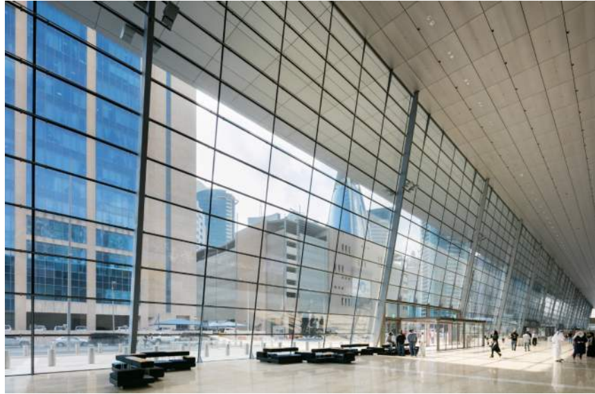
Figure 6 Doha Exhibition and Entertainment Centre – 18m tall horizontal cable facade.
