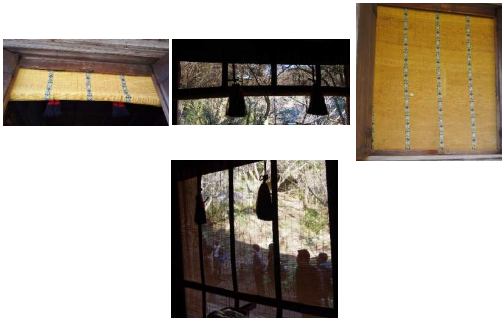
Figure 1: Sudare blind in Japanese traditional building (view from outside to inside and inside to outside)
