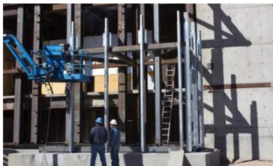
Installation of first floor mullions
