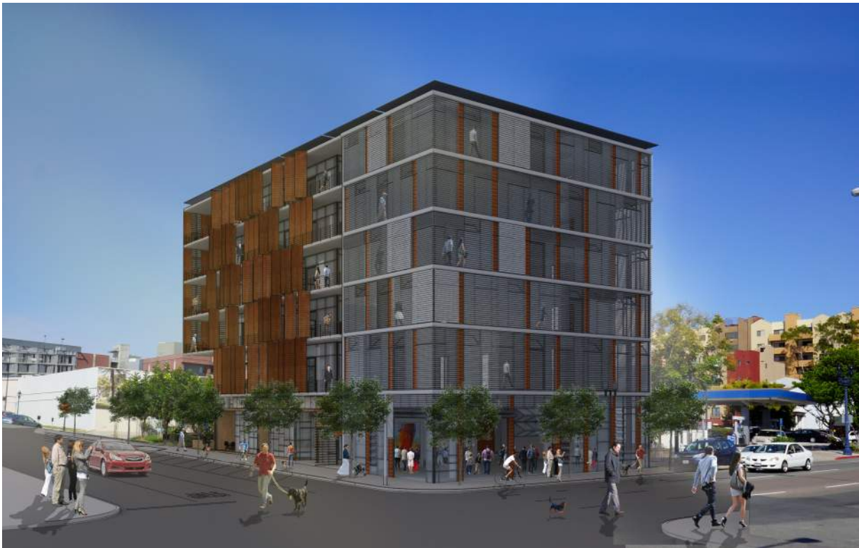
Figure 2 shows a view of the speculative office building from the northwest (top) and the Southwest (bottom). This view shows the sliding operable panels and the exterior venetian blinds. (Drawing by Christianne Jordan)
