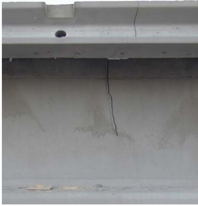
Figure 6-3: Cracking observed during casting, which runs from the deck to the neutral axis [9].
