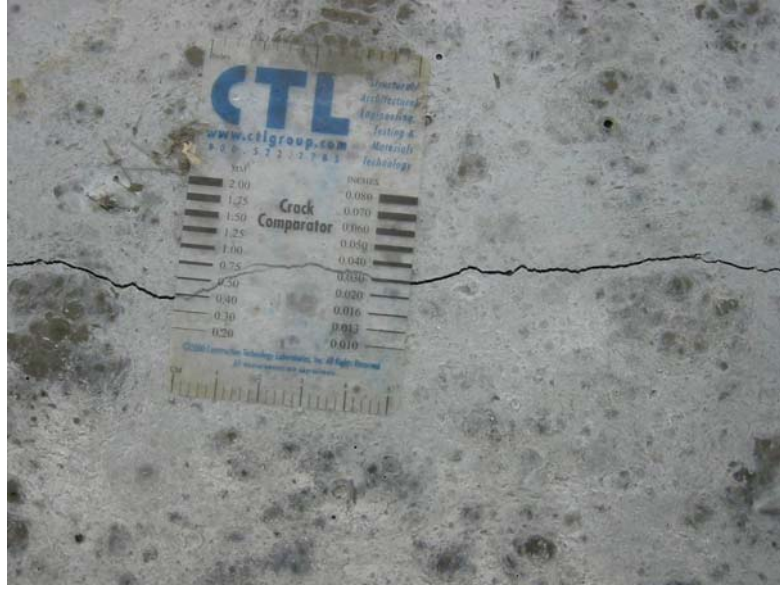
Figure 1-3: Early-age cracking observed during casting of on UHPC bridge girder [9].
