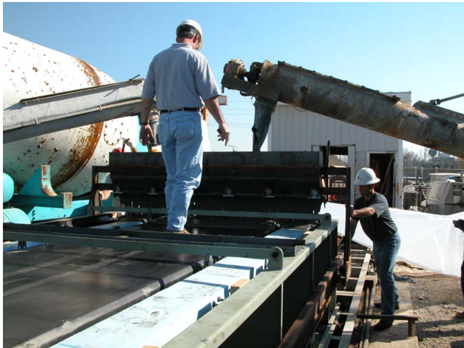
Figure 1-2: Construction of the Ductal TM bridge girders at Lexington, Kentucky [9].
